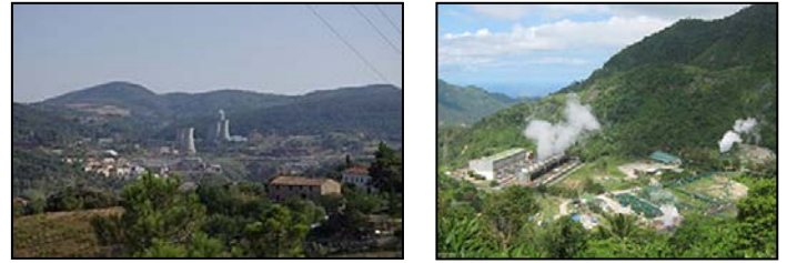
Fig. 7 – Geothermal power stations: a) Larderello, Italy, b) Negros, Philippines
